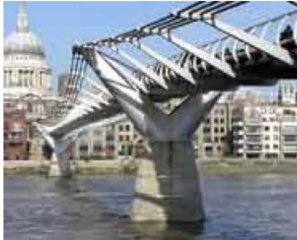
The London Millennium Bridge seen from the south bank of the Thames. (Credit: Photo by Adrian Pingstone, courtesy of University of Bristol)
